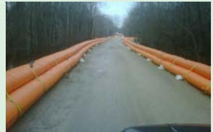
Bladders filled with water are another faster alternative to a sandbag barrier. -From U.S. Flood Control, makers of "Tiger Dams."
