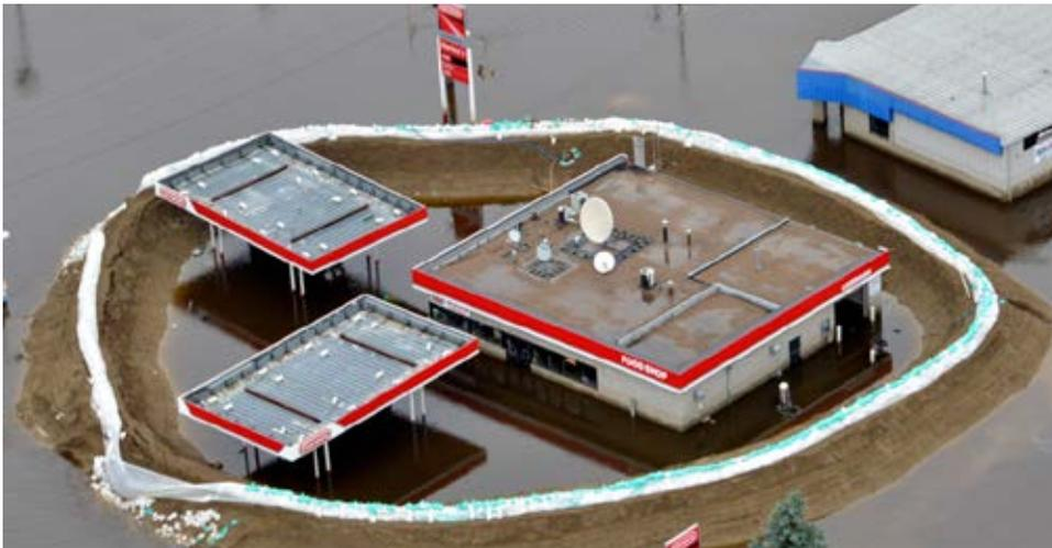
Critical facilities managers need to understand that permanent mitigation measures are better than relying on emergency flood fighting. This gas station had an emergency ring dike that either leaked or was flooded by subsurface percolation. Minot, ND 2011. -FEMA Photo by David Valdez
